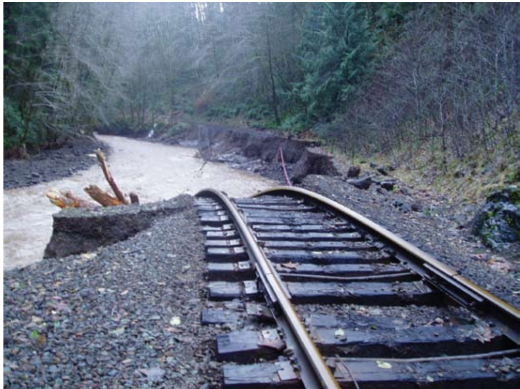
Floodwaters washed out a rail line in the Pacific Northwest during the destructive December 1-3, 2007 winter storms that pounded the Pacific Coast. Credit: National Weather Service
